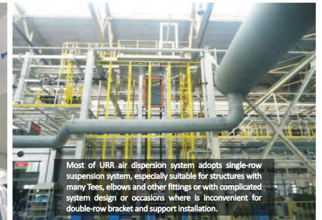
Most of URR air dispersion system adopts single-row suspension system, especially suitable for structures with many Tees, elbows and other fittings or with complicated system design or occasions where is inconvenient for double-row bracket and support installation.
