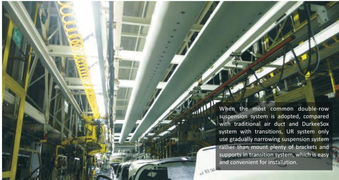
When the most common double-row suspension system is adopted, compared with traditional air duct and DurkeeSox system with transitions, UR system only use gradually narrowing suspension system rather than mount plenty of brackets and supports in transition system, which is easy and convenient for installation.
